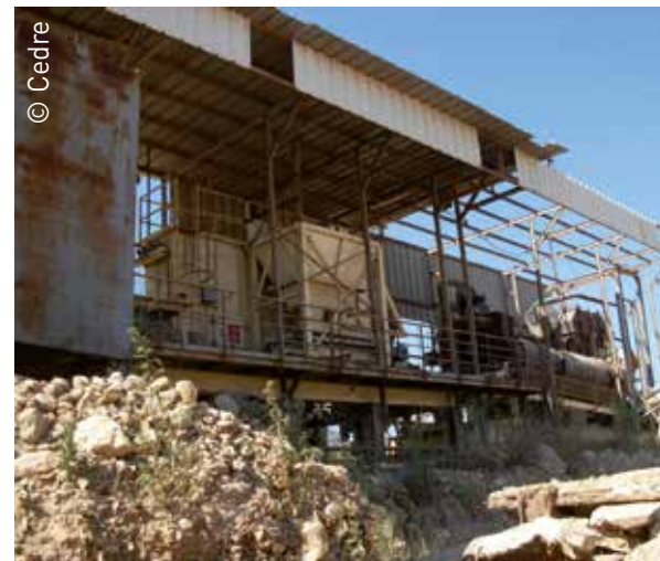
Thermal desorption equipment on site
